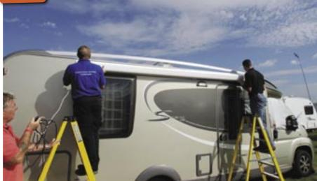
At this stage, the awning is test-fitted and the wiring connections planned. The 12V electric motor for the awning is at the left hand end of the awning, but wiring connections had to be made at the right hand end of the unit - a channel behind the awning case hides the wiring.
