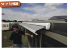
With all the 12V wiring connections made, the operation of the electric awning is checked before all the internal panels are replaced. Once everyone was satisfied with the operation the cables were fied up, the debris from drilling vacuumed up and all the panels replaced.
