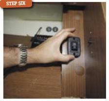
The position of the actuating switch was worked out next and handily the power to the control panel over the door ran through an overhead locker. So the switch could be entirely hidden inside a locker.
