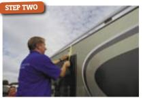
Getting the position of the aluminium brackets correct is vital, so a great deal of time was spent carefully measuring, marking and aligning the three brackets. The exterior light, rear window, side door and the shower cubicle on the driver's side all determined the positioning of the brackets.
